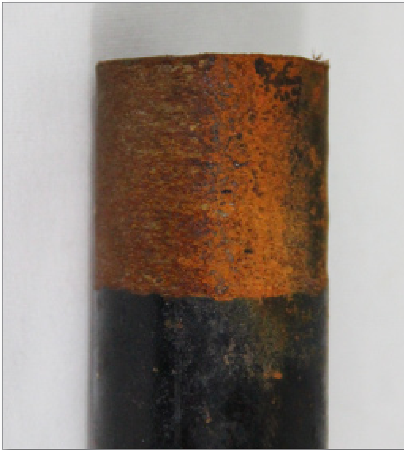
Unprotected metal pipe
